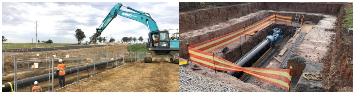
Sydney Water Trunk Main Client: LENDLEASE | VALUE: $7Mil
